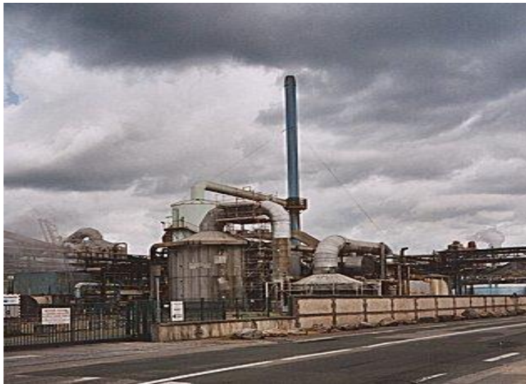
Fig. 1 Reactor A101 of chemical plants
