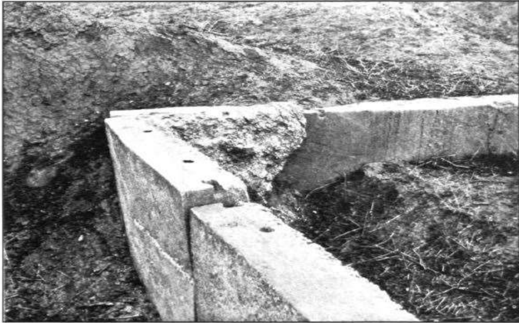
FIG. 61. CORNER OF ROOM IN PALACE OF ASHUR-NASIR-APAL. Note the use of the dowel holes.
